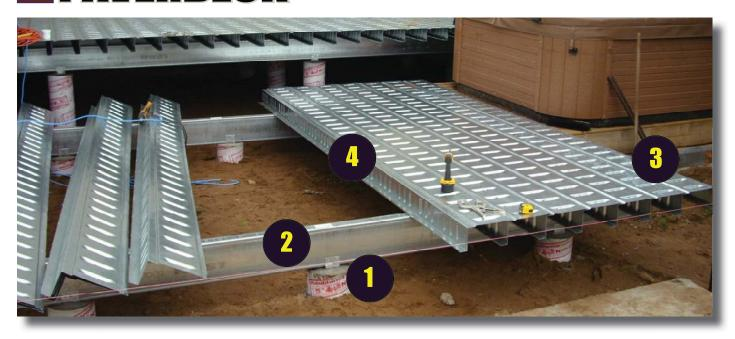
Attach the final End Panel to complete the deck assembly using Tek screws spaced not more than 75.0 mm (3 inches) from the end of the panel and not more than 305 mm (12 inches) between screws. Attach the End Panel to the beam from beneath. If this is not accessible, then you may need to drill a 5/8" hole on the top panel and use a driver extension.
