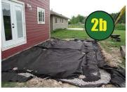
(a) Excavate enough material to bury the beams. Install beams with anodes (optional). and backfill with drainage material. Install decking per the current Paverdeck specification. Slope deck away from house minimum 0.5% to shed water away from house and deck. (b) Consider installing a perforated drain pipe along the perimeter of the deck to carry water away from the footings.
