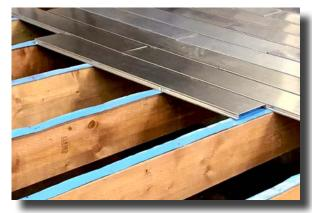
**Screw TILEDECK into joists.**
