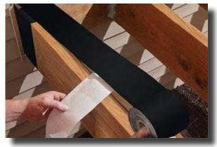
Protect Joists with tape.
