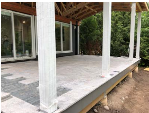
Install tiles/pavers.
